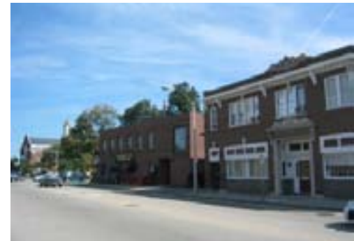
Existing 2-and 3-story Buildings in CBD
