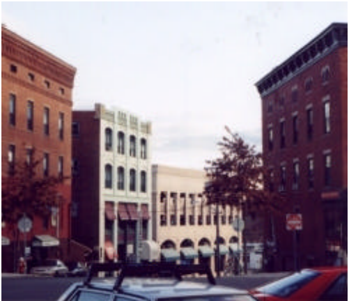
Northampton Parking Garage Nestled Behind Main Street adheres to the Design Guidelines for Building Materials, and Articulation (Detailing).
