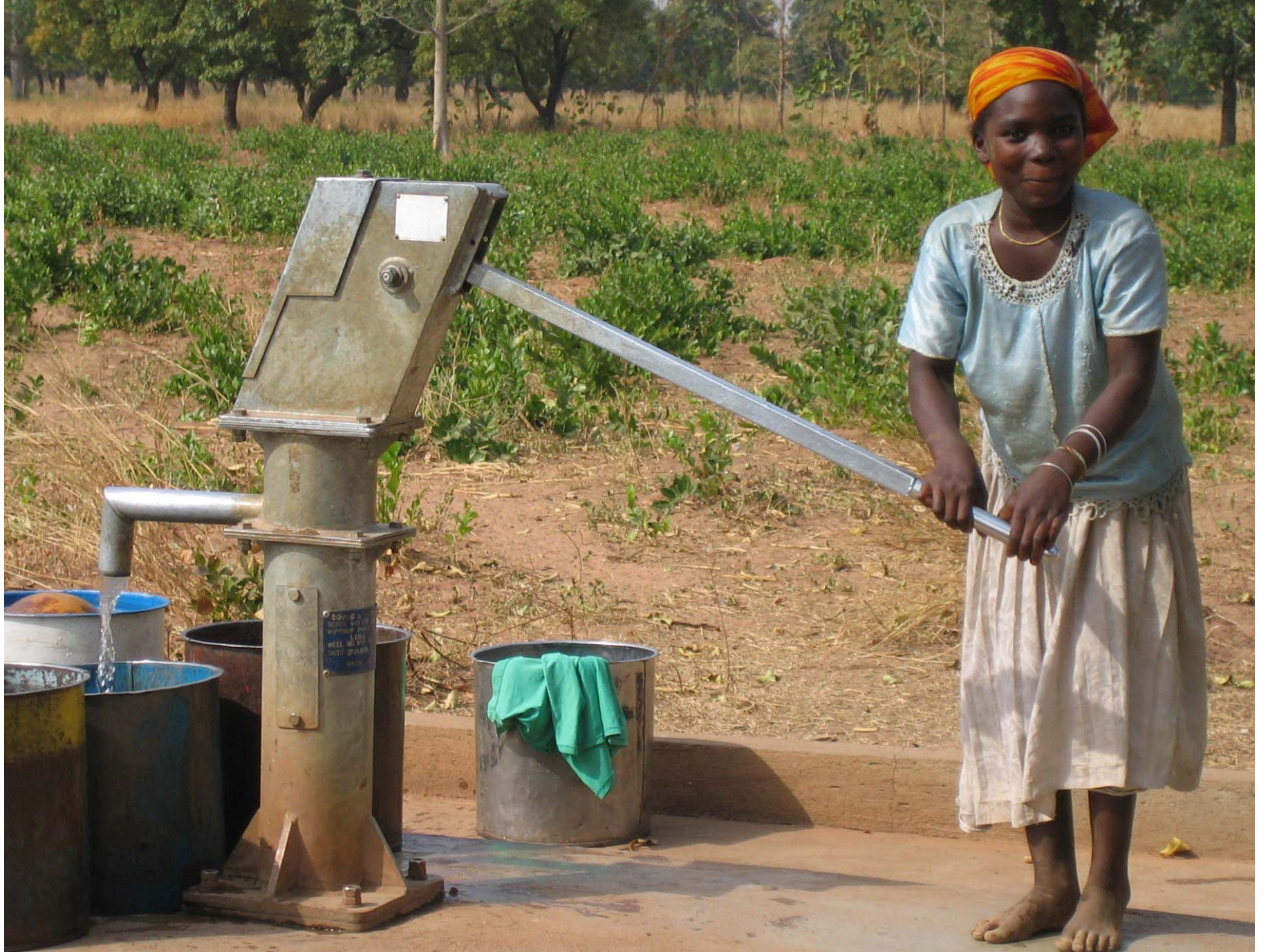
Deep Borehole Well with Lift Pump
