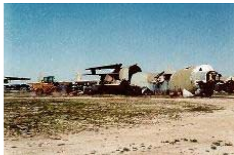
Figure 56. Demolished B-52 with Wings Parallel to Fuselage [24]
