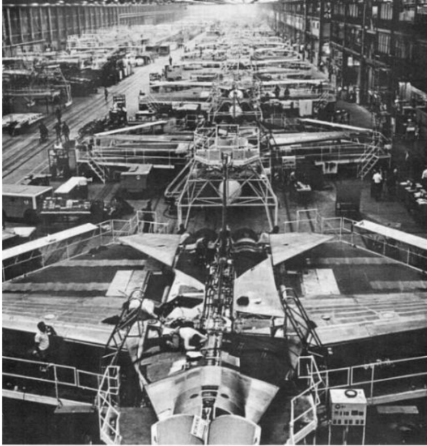
Figure 70: fitting of a wing (from [35])
