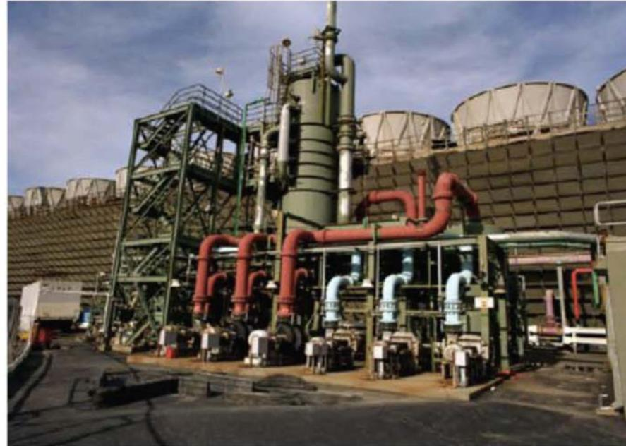
Condensers and cooling towers, The Geysers, being fitted with direct contact condensers developed at NREL
