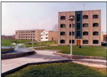
Example of new developments
