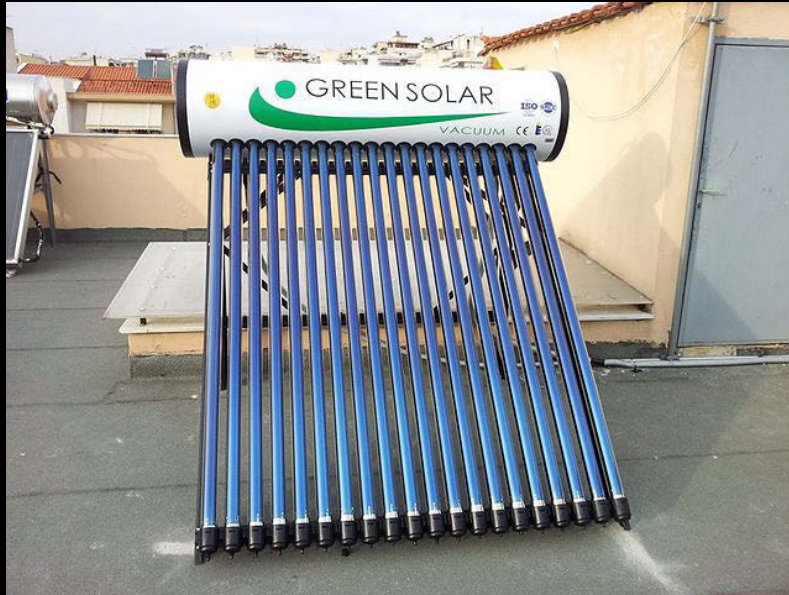
Vacuum Tube Collector. Photo courtesy of Greensolarvacuum on Wikipedia. License: CC BY.
