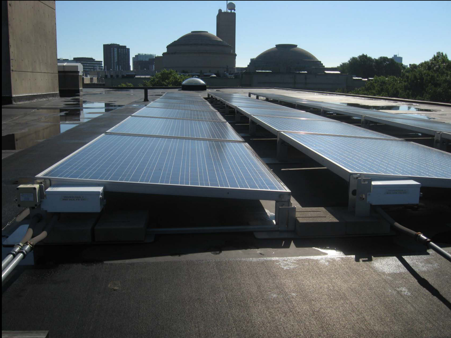
MIT Building W-20, Student Center (Photo courtesy of Alstan Jakubiec. Used by permission.)
