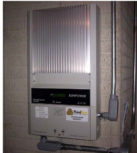
Inverter for Residential PV System Courtesy Prof. Pat Chapman, UIUC
