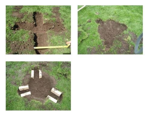
**Figure 3** - Counter-clockwise from top right: Circular dugout with 3 dirt channels, Cross-shaped dugout, and circular dugout with 3 brick-lined channels
