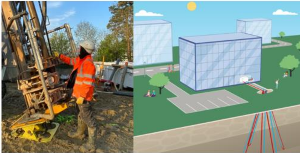
Figure 4 Left: Inclined drilling rig (about 10 degrees) in Paris, France. Right: Simplified illustration of inclined borehole cluster and an accompanying heat exchanger (Celsius Energy).
